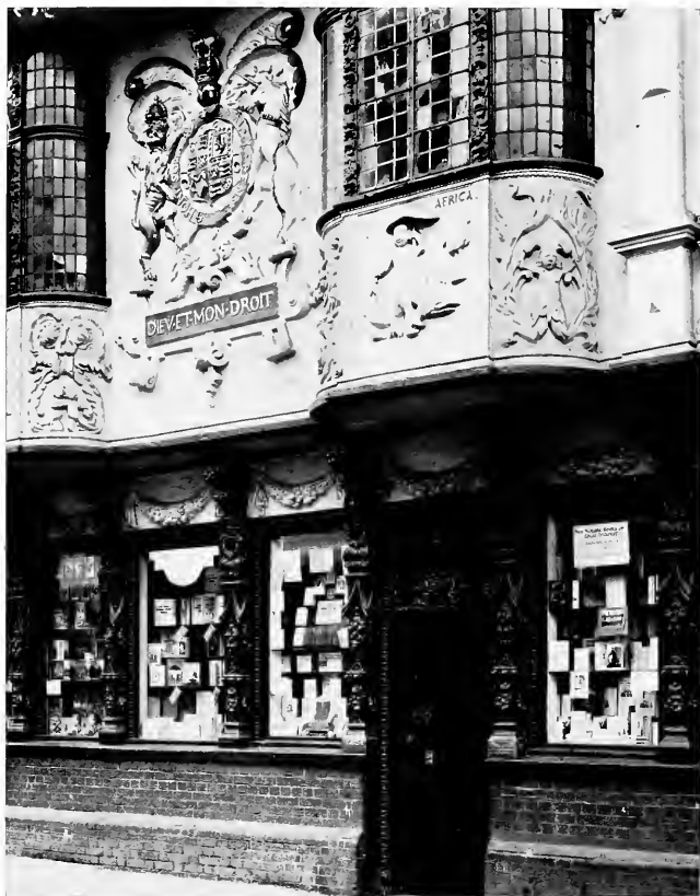
THE ANCIENT HOUSE AT IPSWICH, DETAIL. The finest example of pargeting in England
